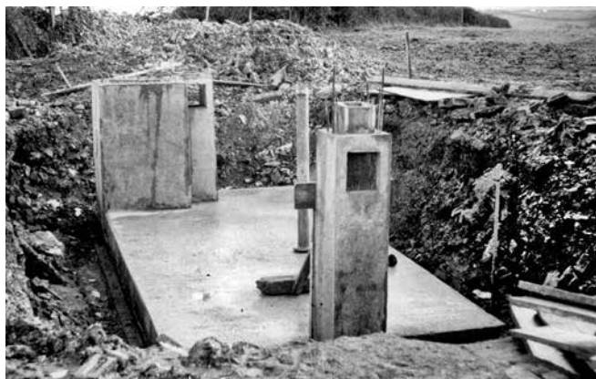
The new bunker almost completed
